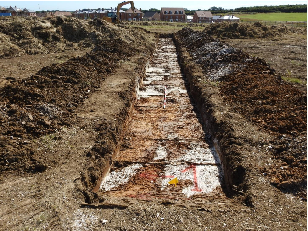
Plate 2: Evaluation Trench 1. Looking east with two metre scale.
